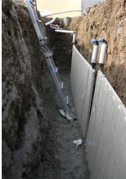
For having the temperature in the soil and in the closed loop, seventy digital thermal sensors are employed in the monitoring system to acquire in real time the temperature; the sensors reach up to 5 m deep in soil, and a density of 1 sensor per  $12 \text{ m}^3$  in the soil surrounding the exchangers.
