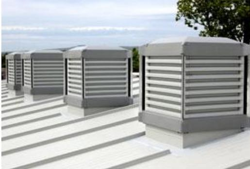
*The Monodraught WINDCATCHER X-Air natural ventilation system is the result of four years intensive research and development, the system bristles with innovation and a number of patented technologies.*
