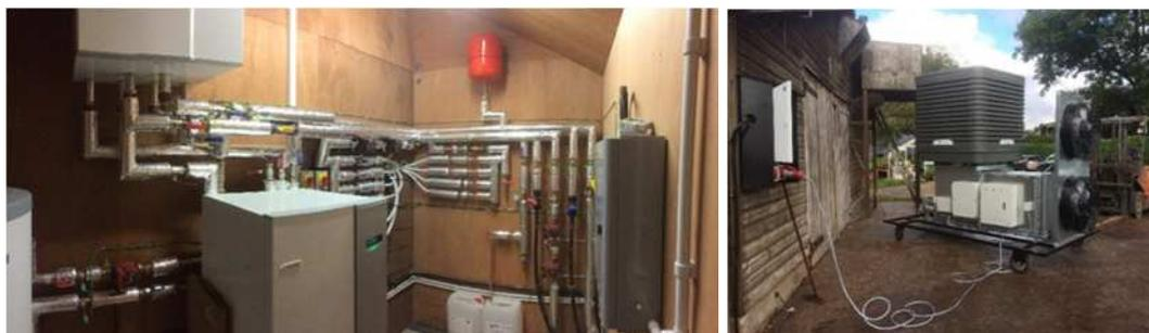
Fig 2 – (a) WelChic heating system plant room containing heat pump, buffer tank & controls, and (b) WelChic PEC cooling system
